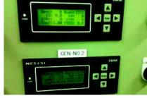
Alternatively the FlexGen controllers can be configured through the user interfaces FlexGen UI and C6250. Instead of mounting it permanently the C6250, in this connection, can be used as practical hand tool for making minor adjustments of systems already put into operation.
